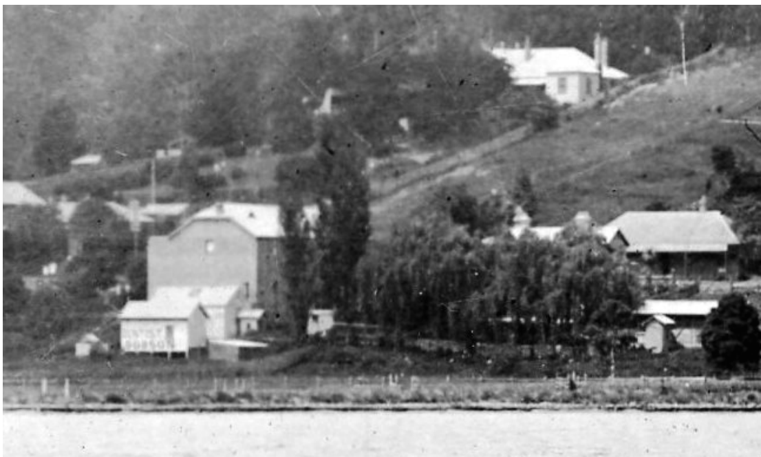
Figure 2.14. This image shows the School of Arts and the roof line of the Police Sergeant's Quarters, together with the outbuildings. It is dated to c.1981. Source: Gosford CC photo collection.
