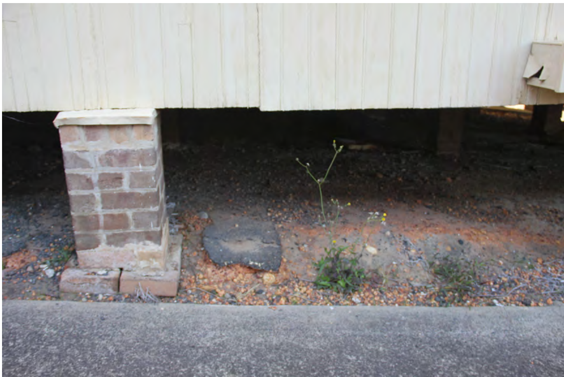
Plates 3.9 and 3.10. One of three timber framed and weatherboarded classrooms on the site. This classroom retains some beaded tongue and groove timber lining and may be dated to the late nineteenth century. The other two classrooms may have been built in the early to mid twentieth century. All appear to have been reused on this site. The building on the Georgiana Terrace frontage is built on brick piers and is likely to preserve the site of the Police Stables beneath. Photograph by Dr. Edward Higginbotham.
