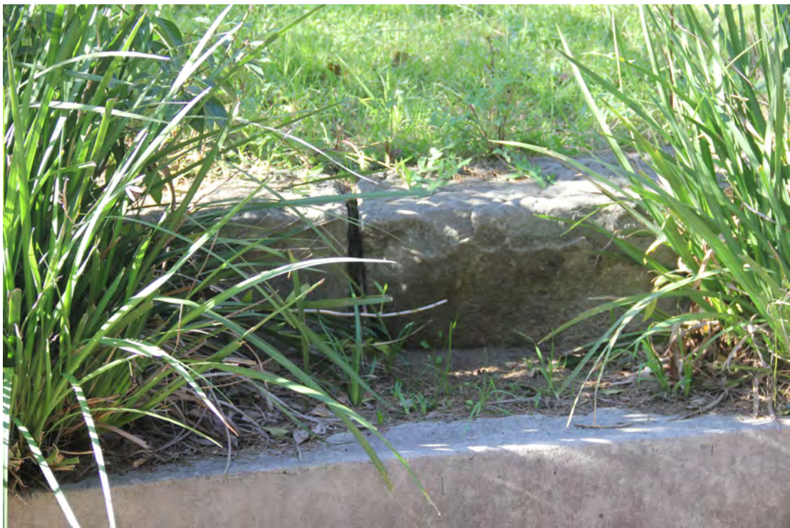
Plate 3.7. Part of a U shaped arrangement of reused sandstone blocks retaining a grassed area adjacent to the footings of the former Police Sergeant's Quarters and timber framed classrooms.
