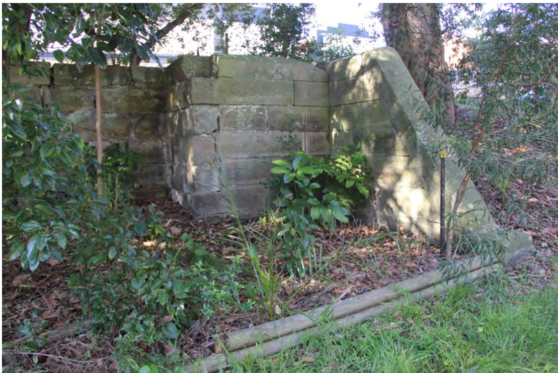
Plate 3.5. The sandstone footings of the retaining wall between the former Police Sergeant's Quarters and School of Arts, fronting Mann Street, Photograph by Dr. Edward Higginbotham.
