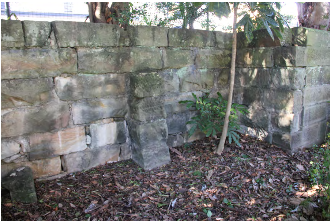
Plate 3.3. The sandstone footings of the former Police Station and Sergeant's Quarters, fronting Mann Street, north-east corner of building.
